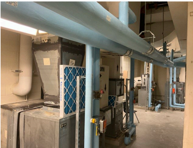
27 - DOMESTIC WATER PIPE
