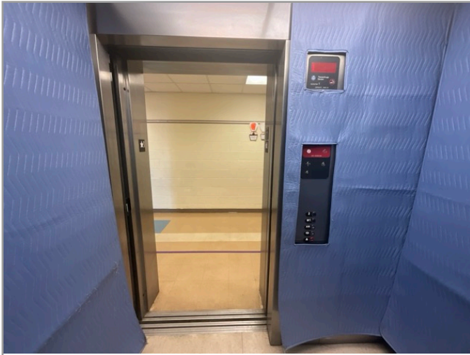
LOBBY LOOKING AT CABS
