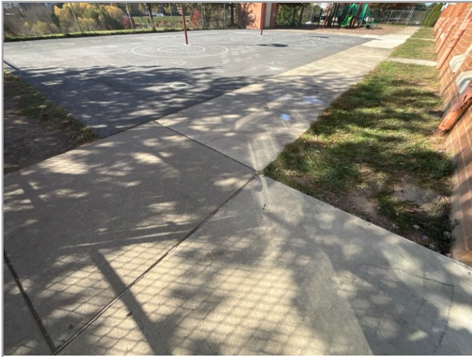
ACCESSIBLE ROUTE TO PLAYGROUND
